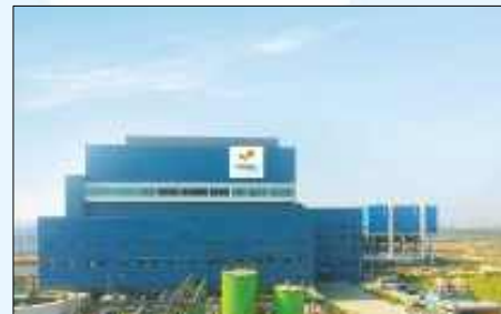
24 MW WTE Plant, Delhi
