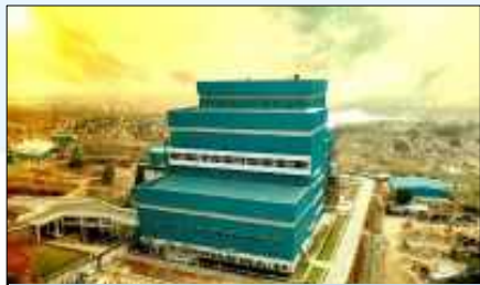
2x600 TPD WTE Power Plant at Hyderabad, TS
