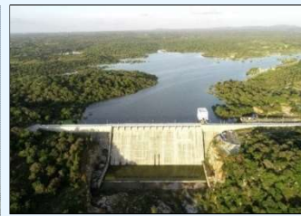
500 Mcft Gravity Dam, Karnataka
