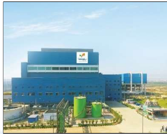
24 MW Waste to Energy Plant, Delhi
