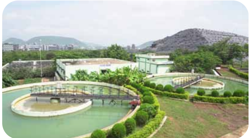
Clarifloculators WTP at Vishaka Energy Limited
