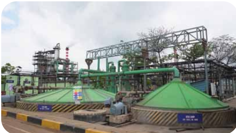
Effluent Collection Sump Selections at Visakha Pharma City Limited
