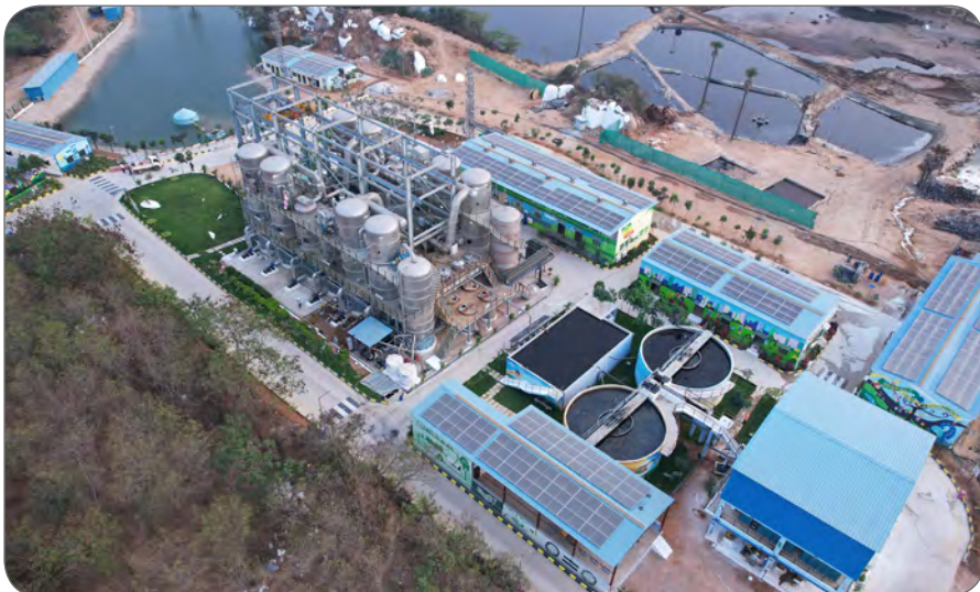
Legacy Leachate Treatment plant at Jawahar Nagar, Hyderabad, Telangana.
